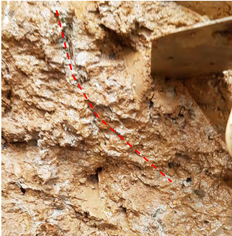
Photo 01: Possible 80 shallowing to 75 degree slip surface in-situ (annotated)
